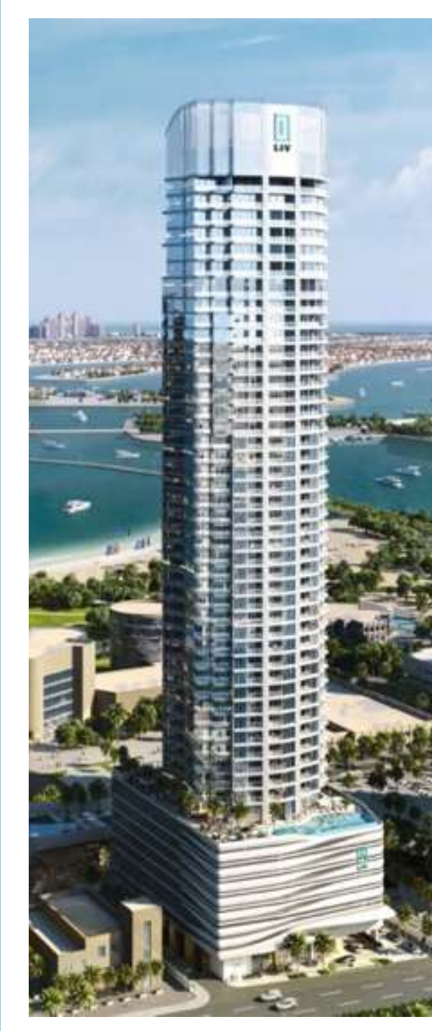
LIV LUX CONSTRUCTION IN PROGRESS HANDOVER 2026
