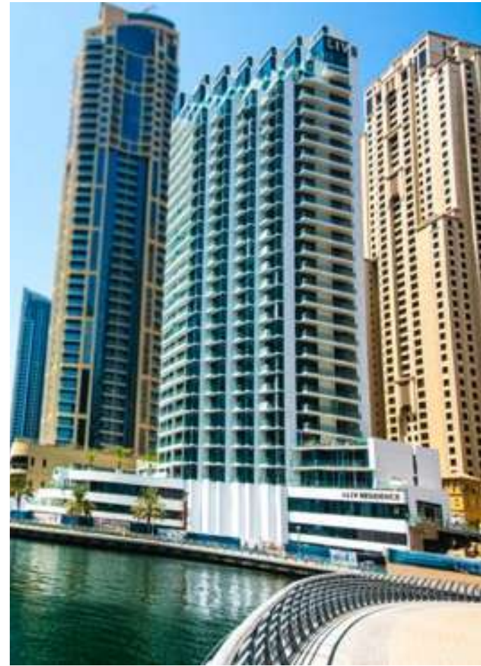
LIV Residence COMPLETED & HANDED OVER
